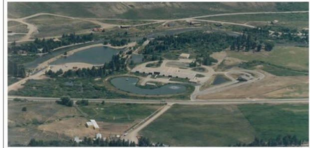
Blue River Wastewater Treatment Plant
