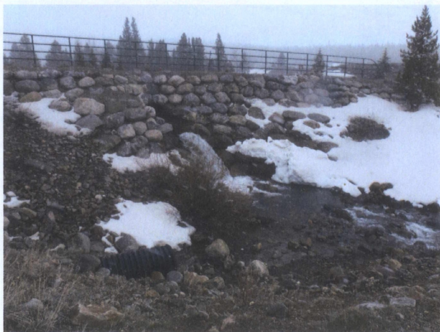
Fish barrier downstream of the Site and WTP.
