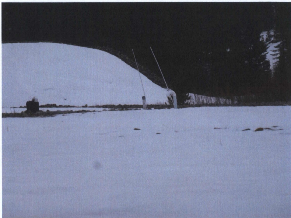
J Pipes indicating discharge location. Treated effluent is discharged below groundwater table.
