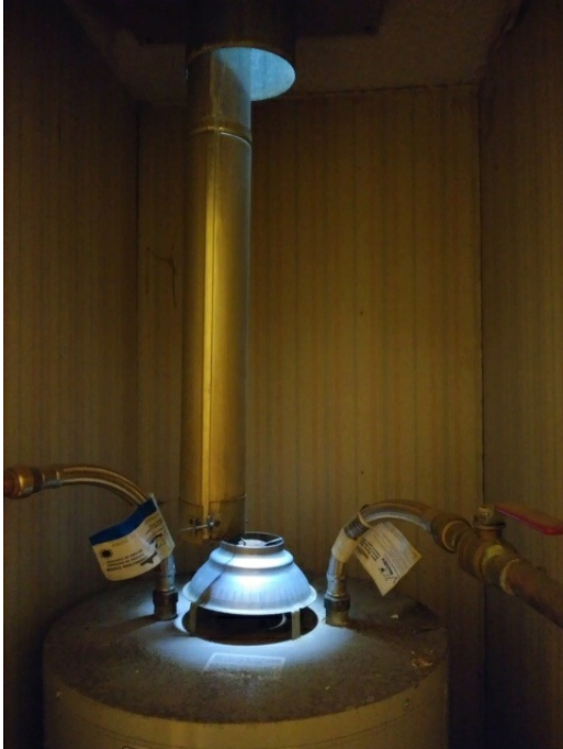
Disconnected flu on water heater
