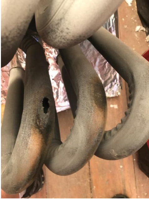
The crack in this furnace caused a serious safety hazard before it was found, and the furnace replaced.
