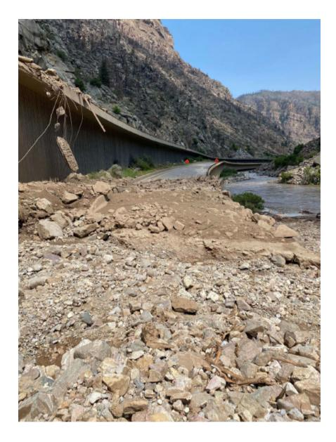
The Glenwood Canyon mudslide damaged much of the infrastructure on Interstate 70, including the Colorado Department of Transportation's fiber-optic cable used to provide service in the canyon.
