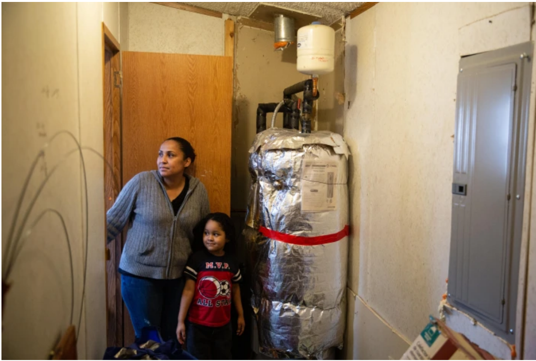
Susana Martinez at her Dotsero, Colorado, home. The Northwest Colorado Council of Governments Energy Program added insulation to her water heater to improve energy efficiency. (Luna Anna Archey, Special to The Colorado Trust)
