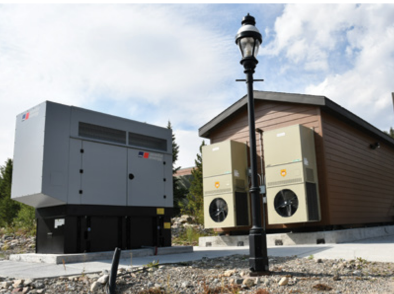
Breckenridge stand-alone Meet-me-Center with air conditioning units and backup power, both requirements for such locations.
