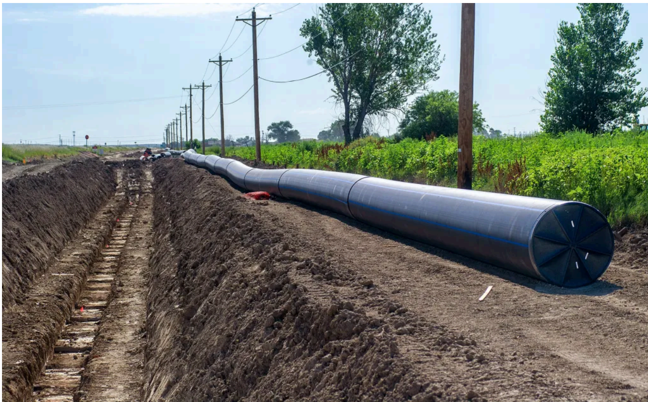
Nearly 1,000 feet of welded pipe lays next to the Arkansas Valley Conduit ditch in eastern Pueblo County. (Mike Sweeney, Special to the Colorado Sun)
