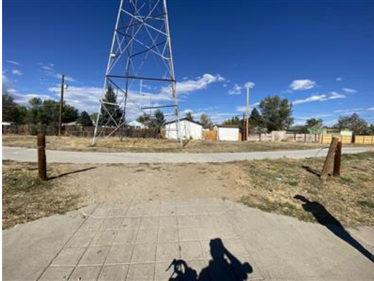
Tennessee Ave Shared Use Path: Gap between curb cut and shared use path
