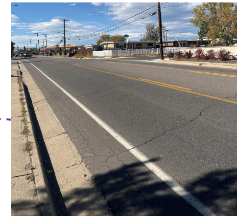
Florida Ave: Current roadway cross section (and center turn lane) leads to high vehicle speeds and a narrow bike lane
