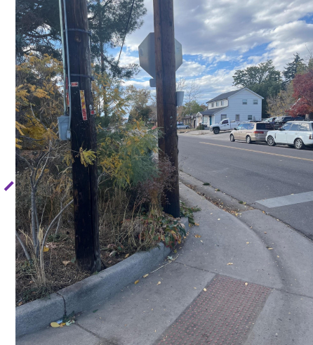
Louisiana & Clay: Obstructed intersection sightline creates a dangerous crossing
